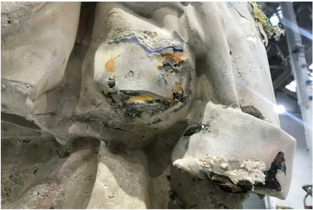
In-progress detail of ...
