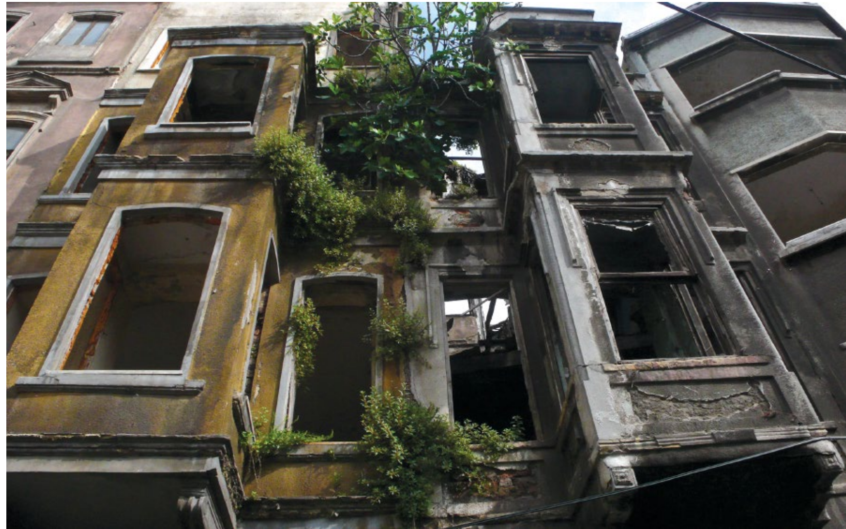
Gregory Buchakjian, photograph of Istanbul's Tarlabaşı neighborhood that was due to be demolished. May 6, 2013, a few weeks before the Gezi Park demonstrations started. Courtesy of the artist.
